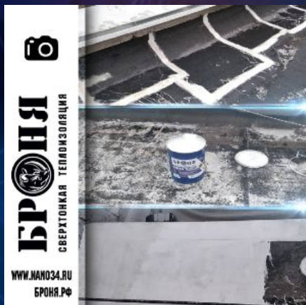
Rubber waterproofing BRONYA AquaBlock Expert in the overhaul of the roof of an apartment building, Ulyanovsk
