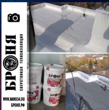
BRONYA AquaBlock in overhaul on the roof of the house, Ulyanovsk
