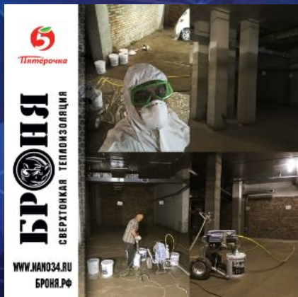
BRONYA Facade for thermal insulation of parking for the Pyaterochka store, Samara
