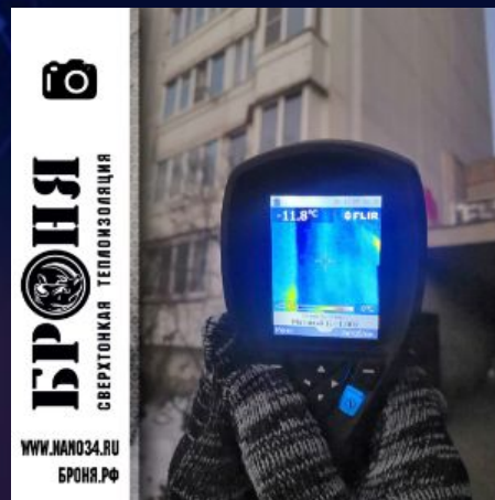
Thermal imaging measurements of BRONYA Facade and confirmation of efficiency in the overhaul based on the temperature difference "before and after", Kostroma
