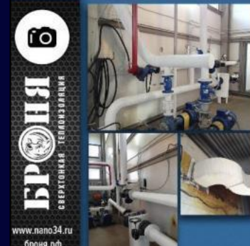
Application of Bronya Classic for thermal insulation of recuperators and steam pipes of the furniture factory "Surgutmebel", Surgut
