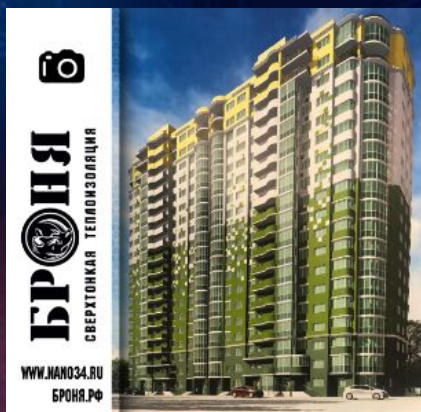
BRONYA Facade during the construction of a multi-storied building "Investradiostroy", Rostov-on-Don
