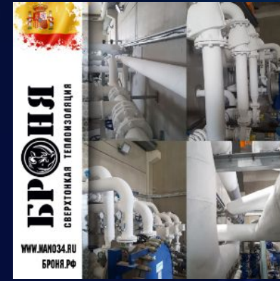
BRONYA Classic on the Aranuez Sewage Treatment Plant Pipeline, Madrid, Spain
