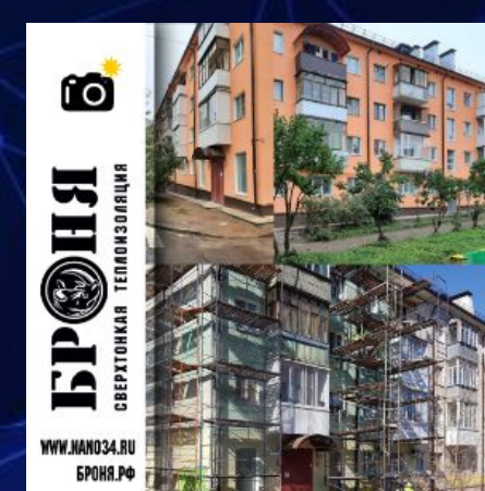
BRONYA Facade NF in the overhaul of a residential building, Smolensk
