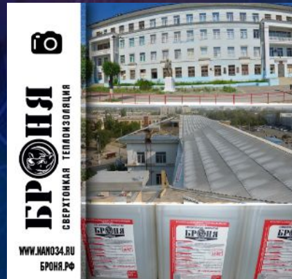
BRONYA Hydrophobizer on the roof of secondary school №3, Opolchenskay a str., 1, Volgograd
