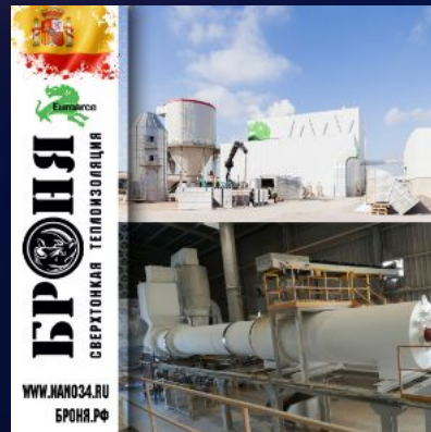
Thermal insulation BRONYA at the Euroace plant in Spain
