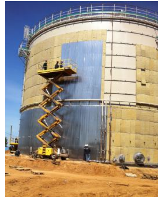
Heat insulation of the reservoir enclosures using mineral wool:
