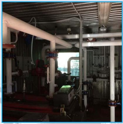
j) Cherepovets, Thermal insulation of the hot water pipeline in the boiler room.
