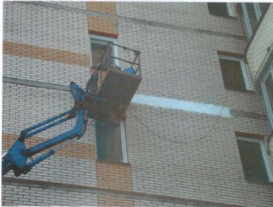
Picture 3. Application of Bronya Winter heat insulation on the butt end of a reinforced concrete floor
