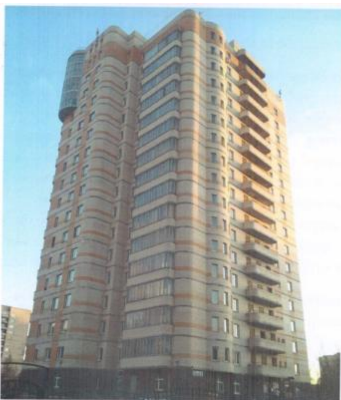
Picture 1. Overall view of the residential apartment building
