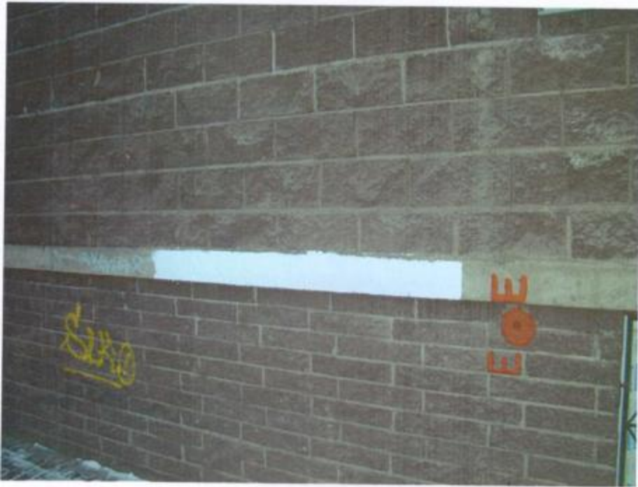
Picture 6. Fragment of the building socle with Bronya Winter heat insulation applied
