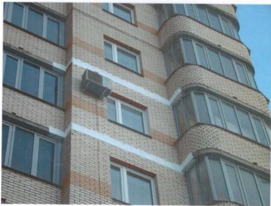
Picture 5. Fragment of the building facade with Bronya Winter heat insulation applied
