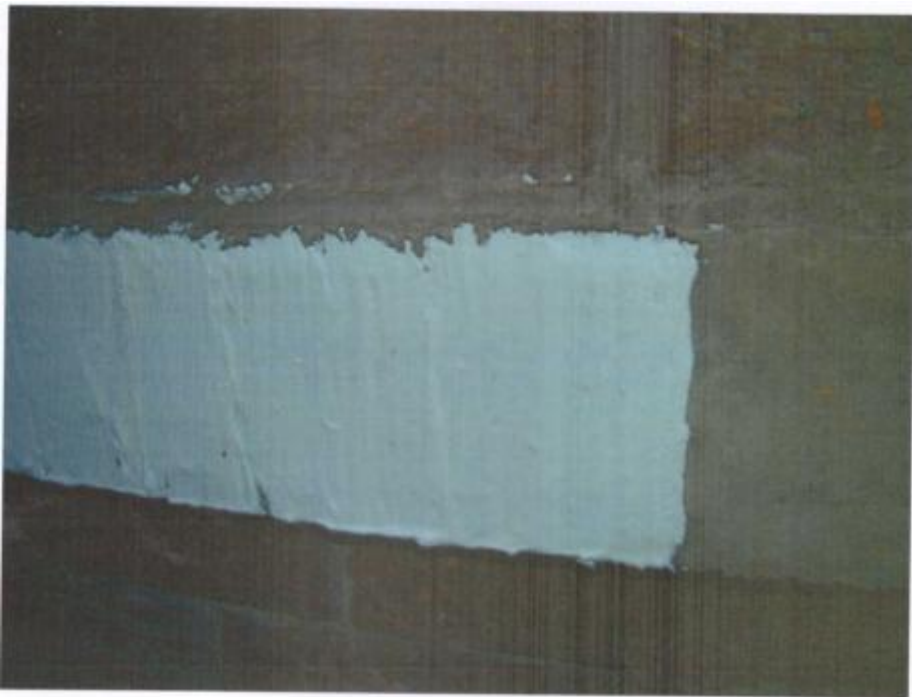
Picture 7. Fragment of the building socle with Bronya Winter heat insulation applied
